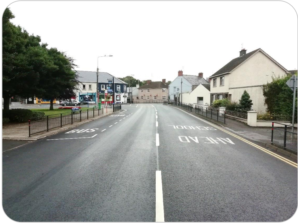
Figure 6 – Drogheda Rd (view to north into junction with R170)
